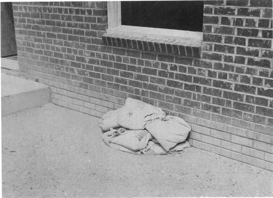
Fig. 2.22 — Sandbagged basement window well.
